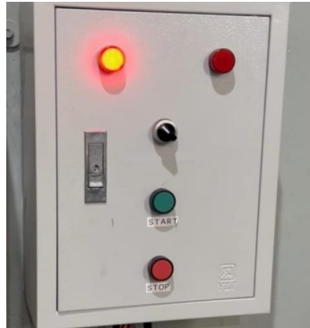
Gambar 3.3 Panel kontrol mesin diesel black start
