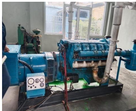
Gambar 3.4 Mesin diesel black start
